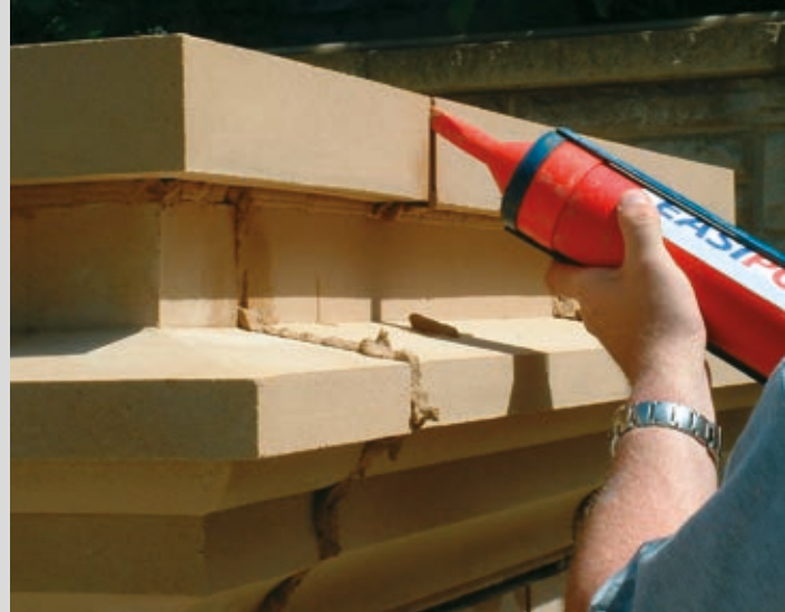
Easipoint mortar during installation.
